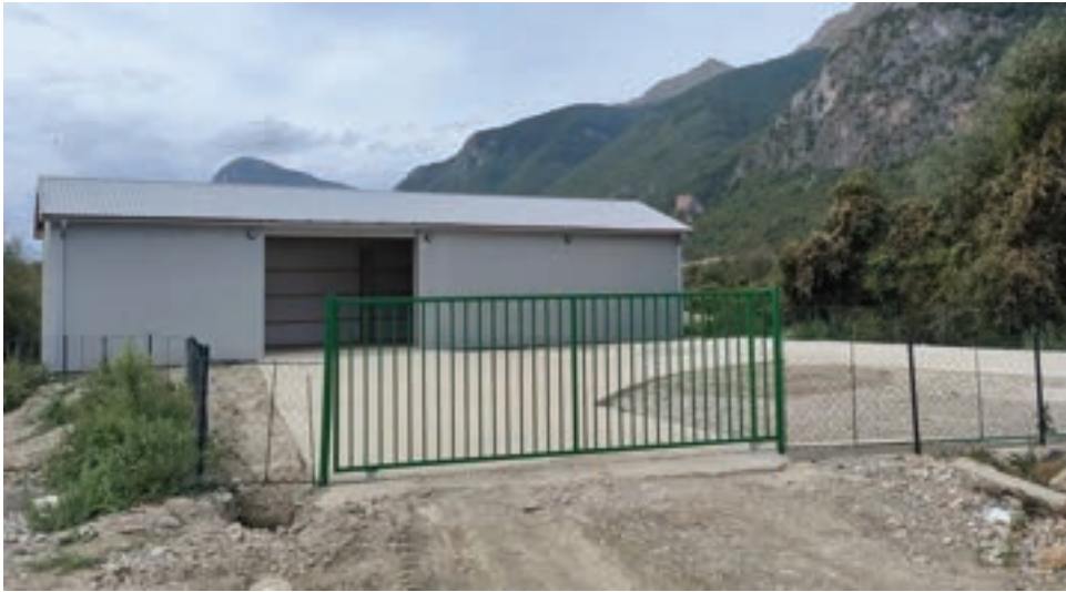
The newly built MRF in Gusinje, ready to receive recyclables
